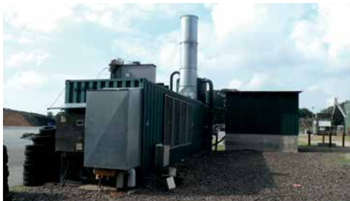
Figure 1. The containerised dryer. The front metal box contains the fore- and back-run pipes of the CHP. Behind the stack on top of the container: the buffer tank for raw digestate
