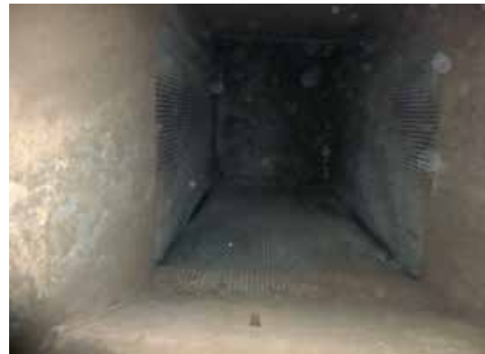
Figure 3. Furnace after a 12-week traveling period with the Shock Pulse Generators installed in 2011
